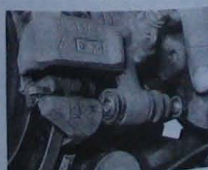
14.8 Pivot the caliper down over the pads and refit the mounting bolt (arrowed)
