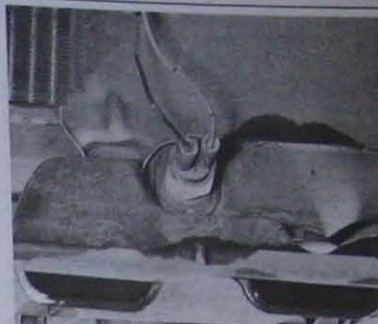
32.30 Water temperature switch location
