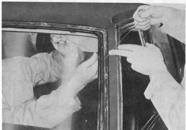
Fig. 14-18 Cutting sealant
